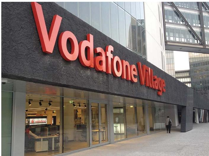
The 27.000 m<sup>2</sup> window area ensures not only bright, light-flooded work stations, but it's special material characteristics regarding energy efficiency significantly reduce the energy requirements for the air-conditioning of the rooms during the summer months. All in all the whole facility, which's concept is strongly oriented on environmental protection, reduces the CO<sup>2</sup> emissions in the area of Milan significant.
